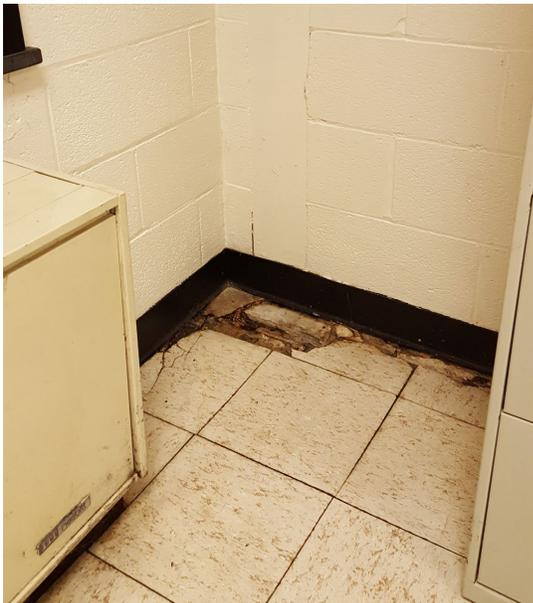
*Cracks and Water Intrusion in the floor*
